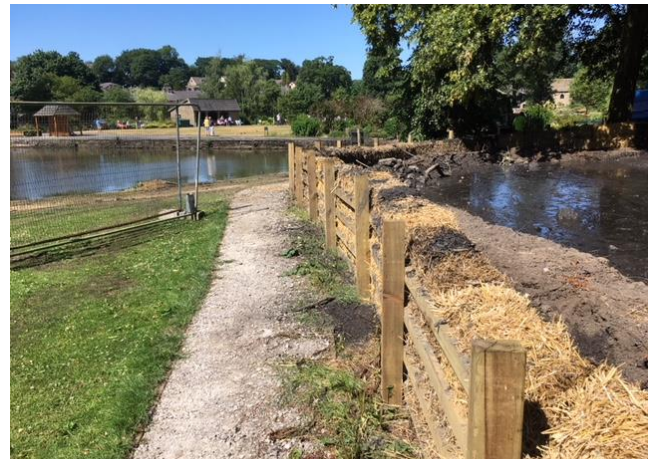
Bund Wall (above); Silt Extracted (below)
