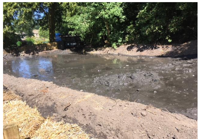
Bund Wall (above); Silt Extracted (below)
