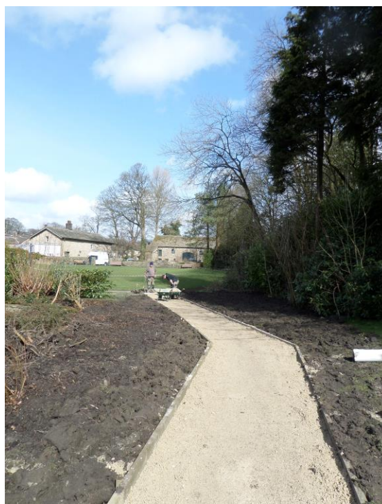
New footpath to rear of Memorial Garden
